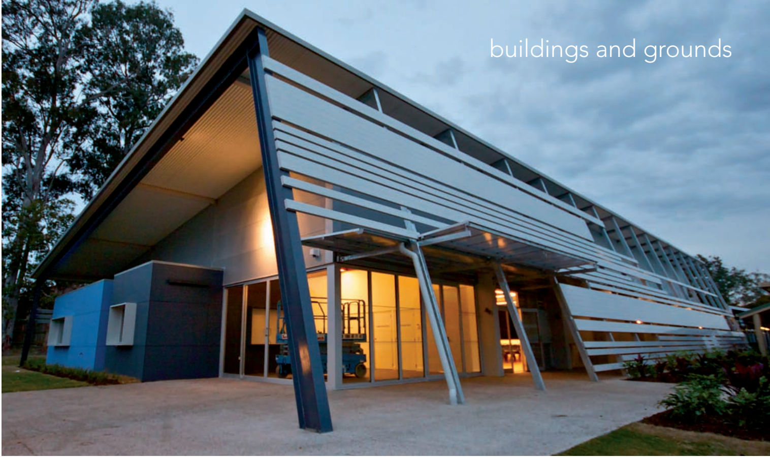
Exterior lighting adds to the atmosphere of evening events at the multi-purpose hall
