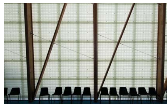
A dual external membrane provides light and contributes to ambient temperature in the school’s hall
