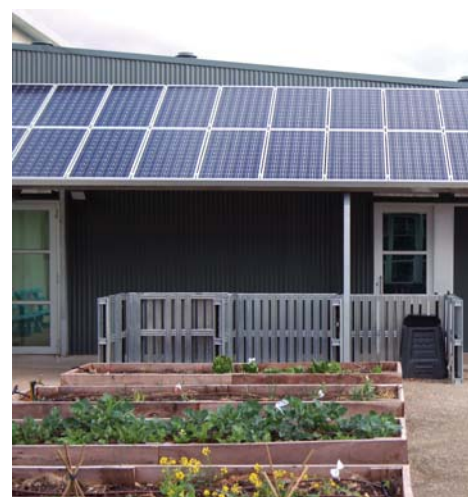
Solar cells double as roofing
